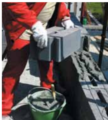
Posa in opera
